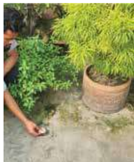
Rooftop Drainage Pipeline
